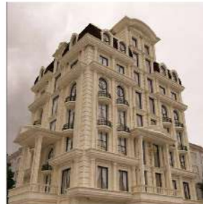
Construction of LaTech, Mashhad, Iran
